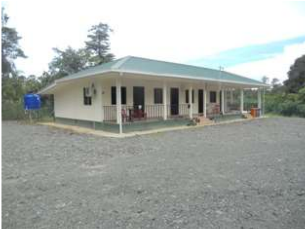
Newly constructed staff quarter at site of FMU 17A forest range office
